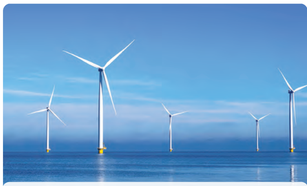
Turbine eoliene offshore (pe mare)
